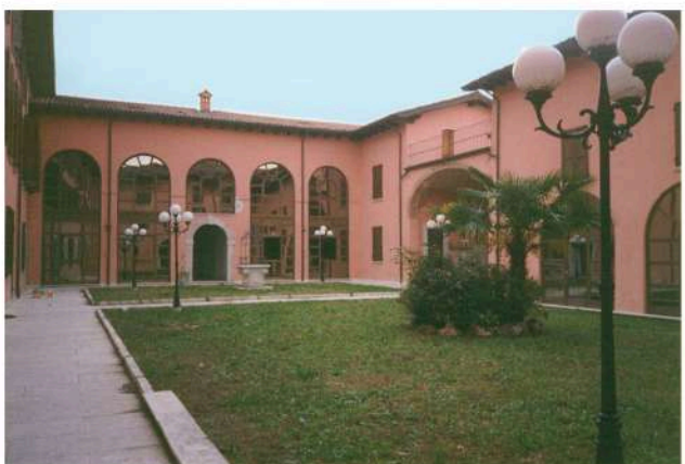
PADENGHE SUL GARDA: FINISHED BUILDING
