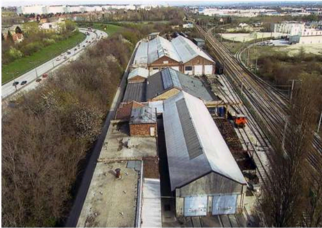
BUILDINGS INSIDE THE PROPERTY (VIENNA)
