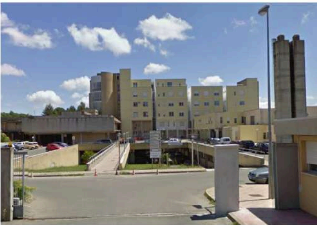
DISTRICT HEALTH CENTRE IN MACOMER
