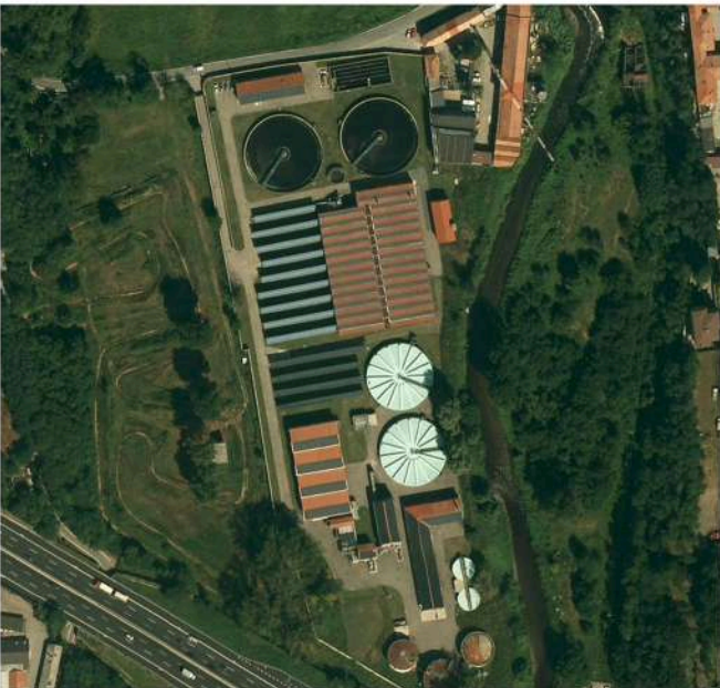
DEPURATOR IN OLGIATE OLONA (VARESE)
