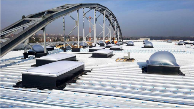
GENERAL VIEW OF THE ROOF
